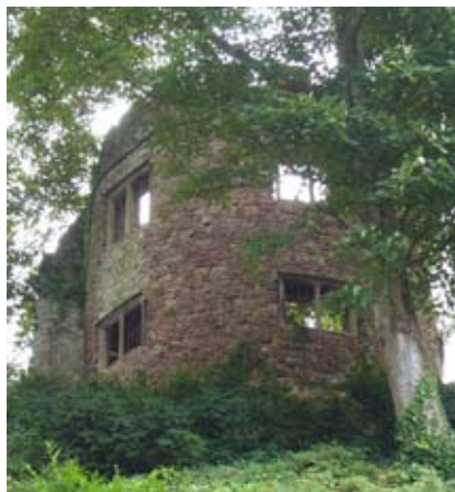
Dunster Curtain Tower
